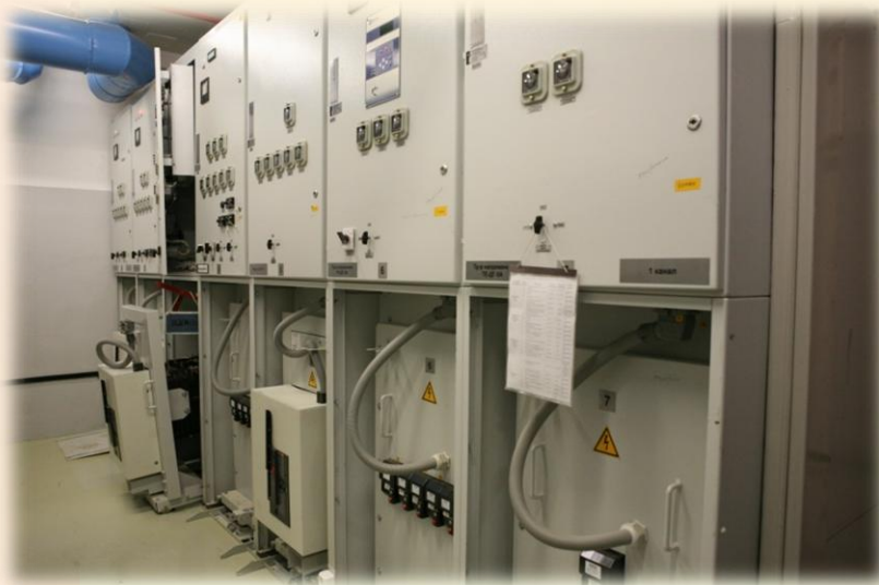
Upgraded power supply system
