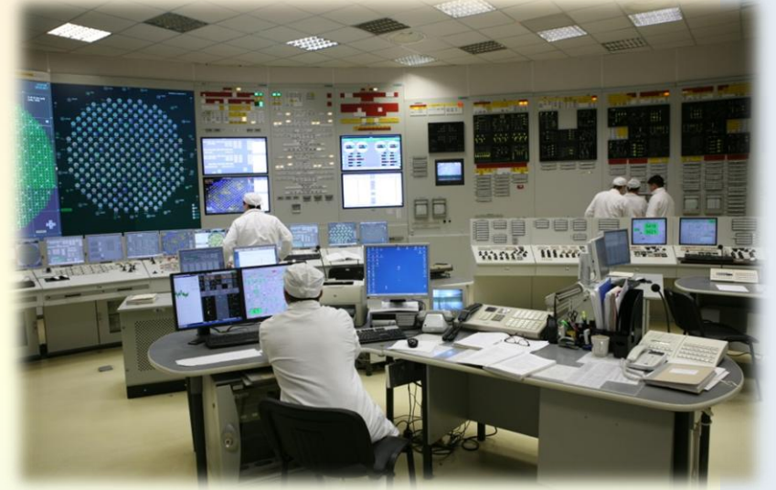
Unit 4 MCR upgraded
