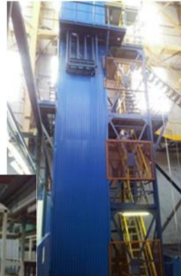
Cell for CRDM test facility
