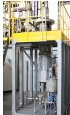
RCP shaft seal mockup test facility
