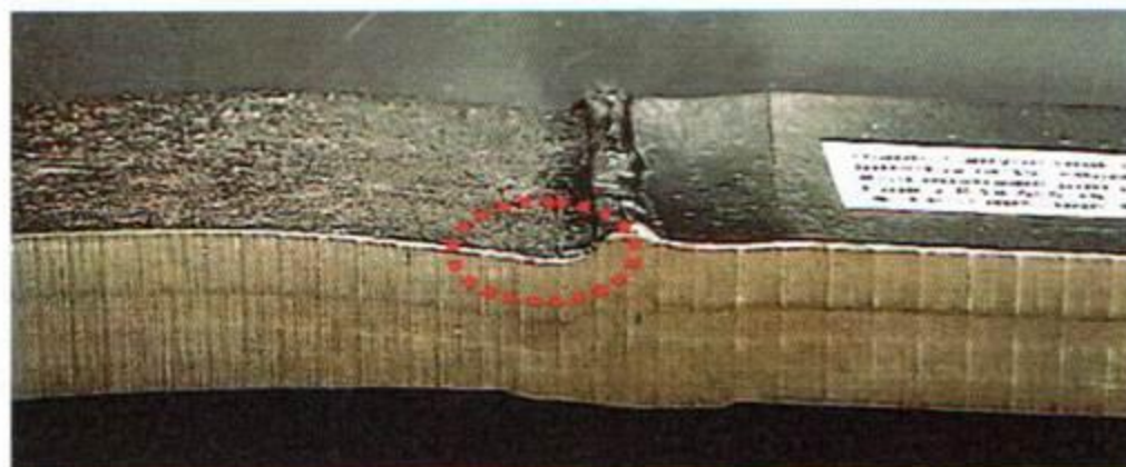
Figure 2 - Close-up of the Weld Shown in Figure 1 (Photograph courtesy of Pacific Gas & Electric)
